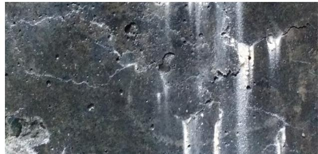
Fig. 8 Crack healing by calcite precipitation
